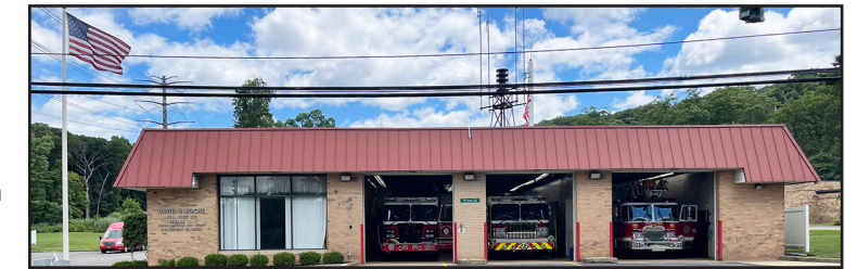
Dangerous overhead high-tension wires, nearly 1 million volts, interfere with ladder testing and use of water for training purposes. Undersized apron creates hazardous conditions requiring the shutdown of US-202 traffic when moving equipment or responding to calls.
